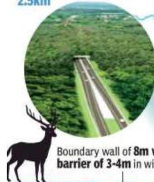
Boundary wall of 8m with sound barrier of 3-4m in wildlife section
